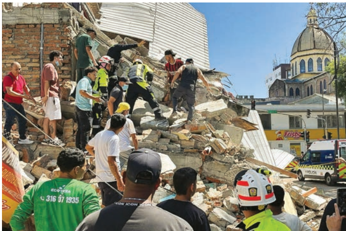
Residents and emergency personnel dig through the debris of a partially collapsed building after an earthquake, in Pereira, Colombia. (Reuters)
