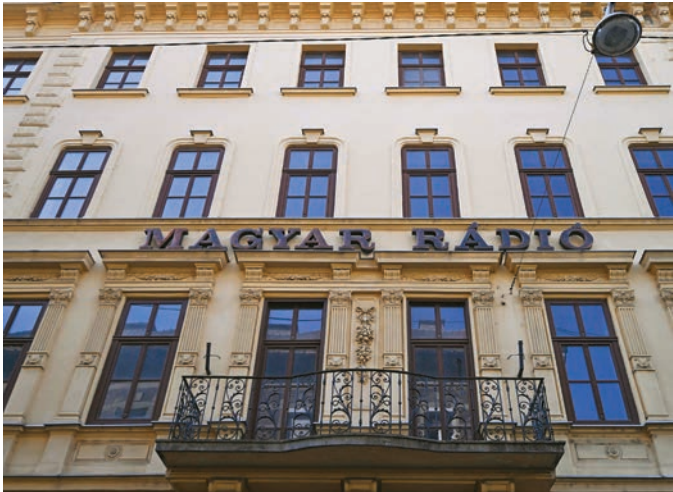
The remainder of facade of the former Hungarian Public Radio building, Magyar Radio in Budapest, after it was demolished. (AFP)
