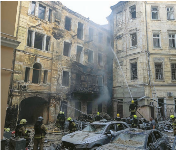
Ukrainian rescuers work in the courtyard of a damaged building at the site of a Russian air attack in Odesa yesterday. (AFP)
