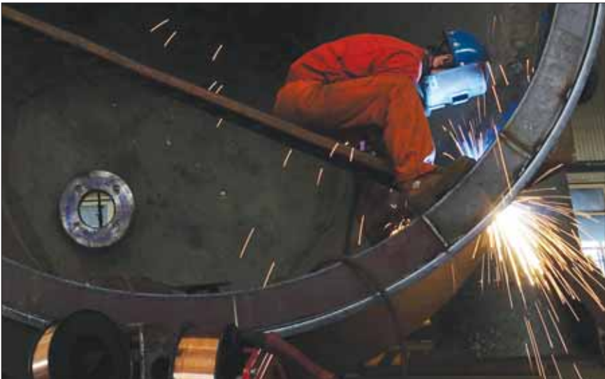
A worker welds a steel structure at a plant in Dalian, Liaoning province. China's leaders, confronting a two-speed economy of strong factory output and exports but weak domestic demand, have pledged to bolster growth by accelerating fiscal spending on already budgeted infrastructure projects through year-end.
