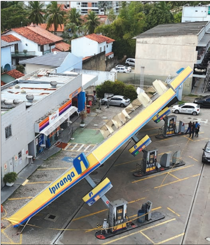
A drone view shows a damaged gas station that collapsed during strong winds in Rio de Janeiro, Brazil, yesterday. (Reuters)
