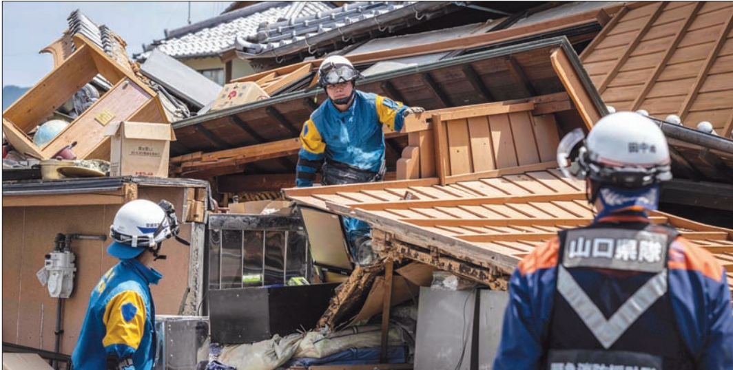
Rescue officials work at the site of a house that collapsed following the earthquake, in Yatsushiro, Kumamoto prefecture, yesterday. (AFP)
