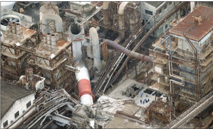
An aerial view shows a collapsed chimney at Nippon Paper Industries' Yatsushiro Mill after an earthquake in Yatsushiro, Kumamoto Prefecture, yesterday. (Reuters)
