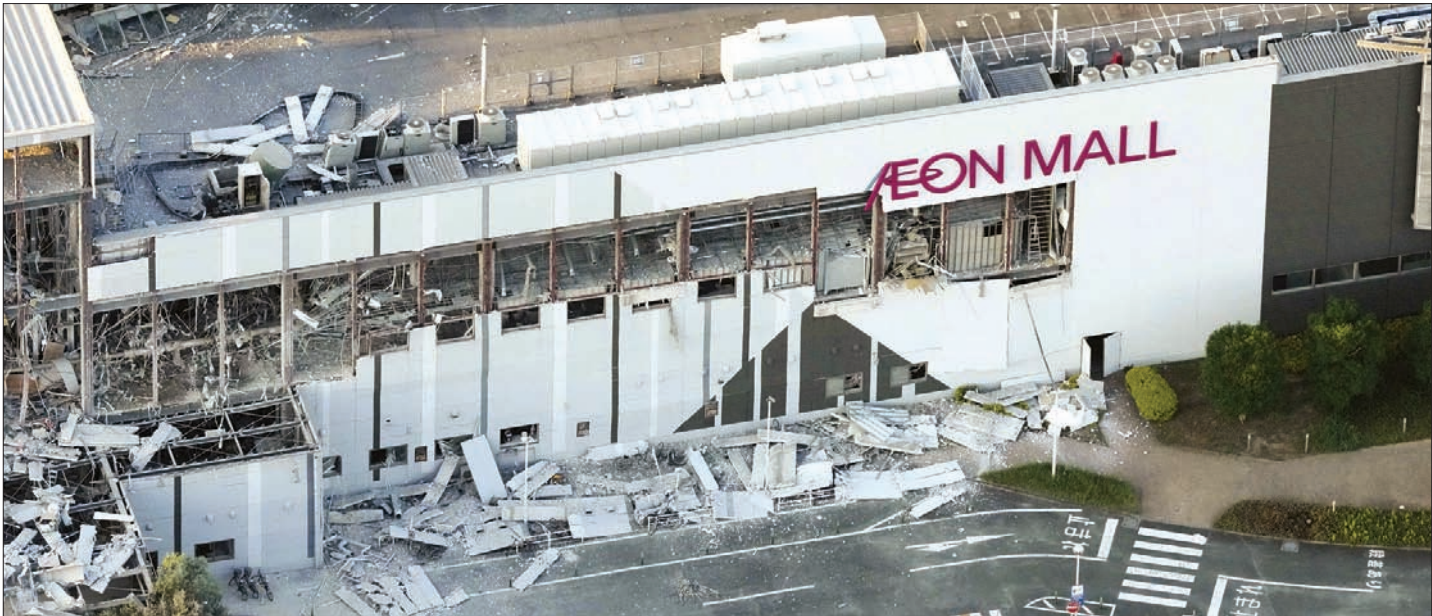
An aerial view shows the damaged Aeon Mall shopping centre, where, according to local media, an explosion occurred after an earthquake with a preliminary magnitude of 7.1 struck Japan’s southern Kumamoto prefecture, in Kashima Town, yesterday. (Reuters)
