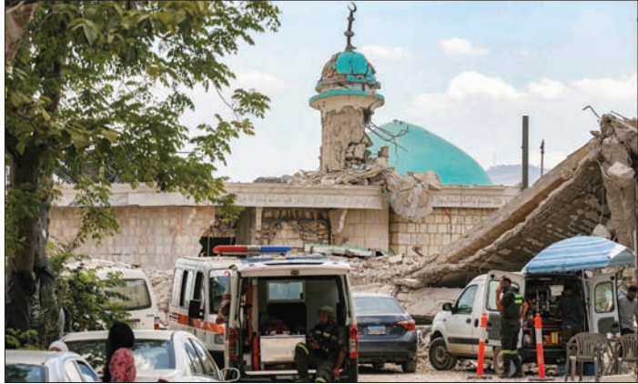
First responders deploy near a heavily-damaged mosque in the village of Zawtar al-Gharbiyeh in southern Lebanon. (AFP) /
