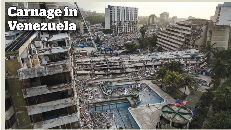
Aerial view of residential buildings destroyed after the earthquake of July 24, in Caraballeda, Venezuela on Monday. The number of people killed in the powerful dual Venezuela earthquakes last month rose to 5,278, according to official figures updated on Monday. (AFP)
