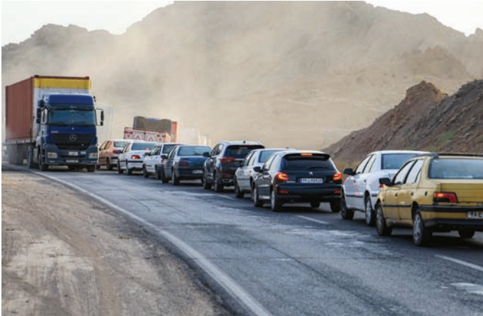
Vehicles wait in traffic near a heavily-damaged bridge connecting Roudan and Bandar Abbas in southern Iran that was hit by US. (AFP)
