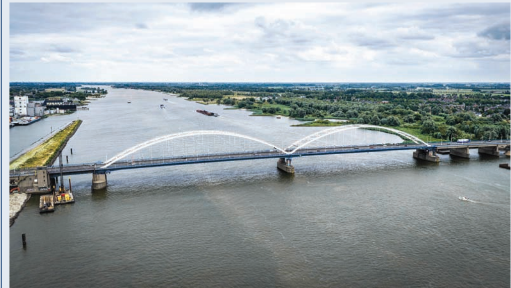
This aerial photograph shows a view of the Merwede Bridge near Gorinchem yesterday. According to Rijkswaterstaat, research shows that the arch structure of the bridge, which carries the A27 motorway, is weaker at multiple locations than previously assumed. (AFP)
