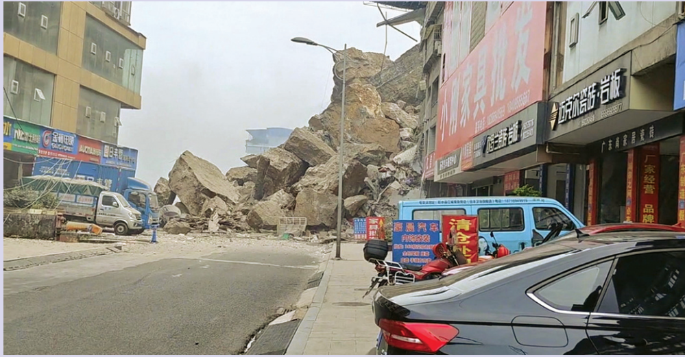
Debris is seen at the site of buildings that collapsed due to a landslide in Chongqing, China, yesterday, in this screengrab obtained from a social media video. (Reuters)
