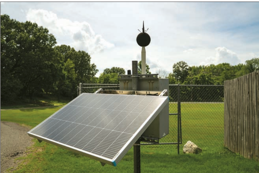
A sound monitoring system in the Colonial Hills neighbourhood located in Southaven, Mississippi. The neighbourhood sits adjacent to xAI's gas turbine facility, where the constant noise of the turbines can be heard throughout the community. (Reuters)
