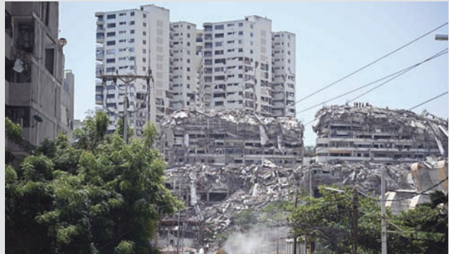
A backhoe removes debris in Catia La Mar, La Guaira state, Venezuela, following twin earthquakes. The death toll from the deadly earthquakes that hit Venezuela on June 14 has surpassed 4,700, while almost 17,000 people have been injured, an official report stated. (AFP)
