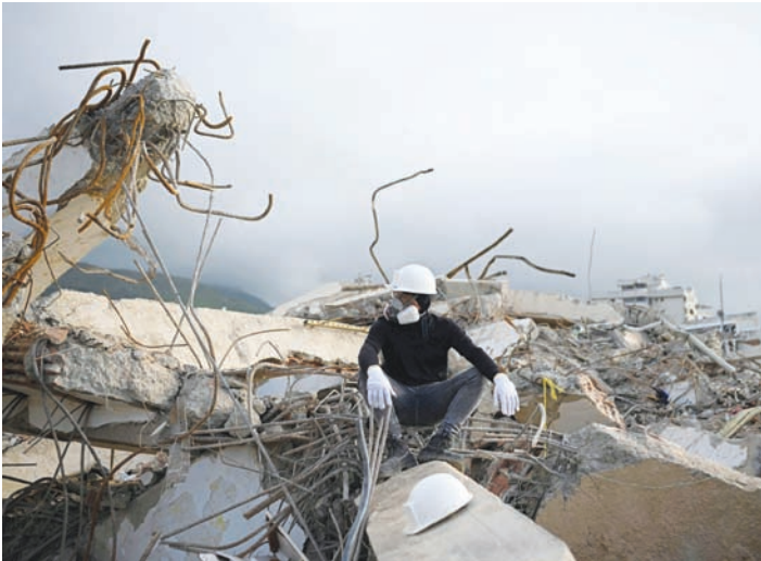
A rescue worker wearing protective gear pauses atop the rubble of a collapsed building in Los Corales, La Guaira state, Venezuela. (AFP)
