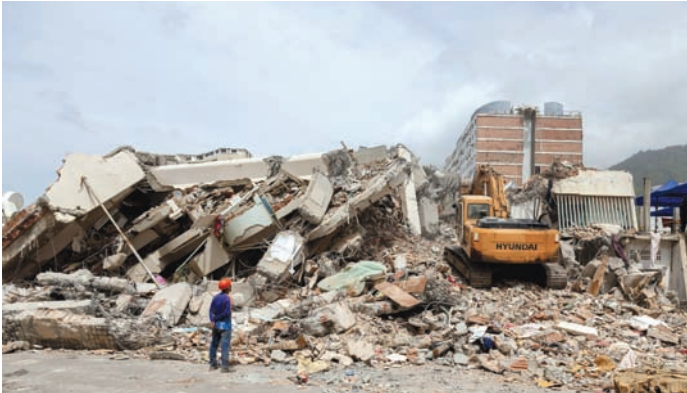
An excavator removes debris from the site where Maria Alejandra Sanz was trapped for 17 hours in La Guaira. (Reuters)
