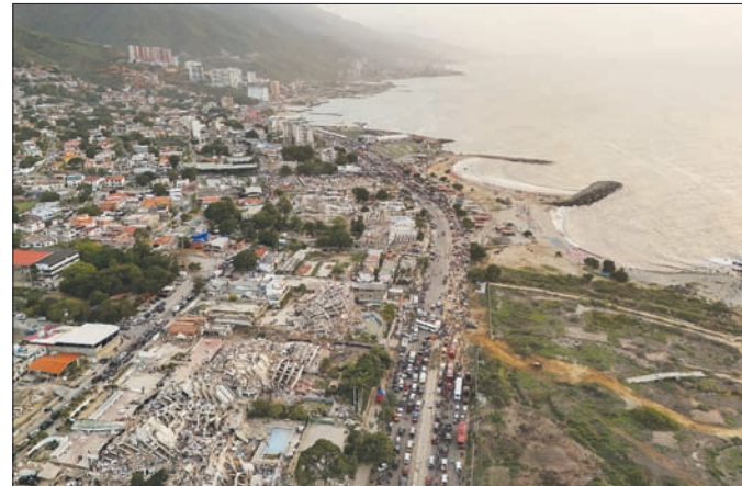
A drone view shows buildings destroyed in La Guaira. (Reuters)
