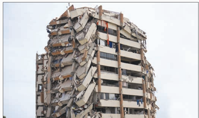
A view shows a heavily damaged apartment building following an earthquake in Catia La Mar, La Guaira state, yesterday. (AFP)
