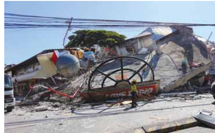
A worker walks near a collapsed building following the magnitude 7.8 quake in General Santos, yesterday. (Reuters)
