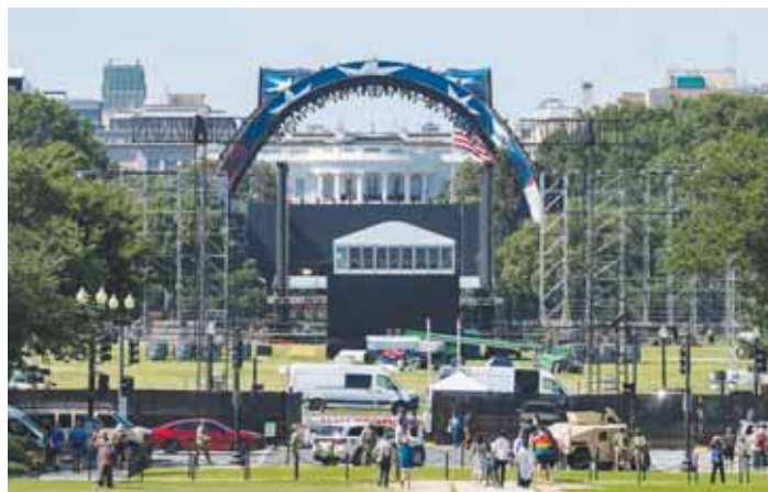
Construction continues for the UFC event. (Reuters/File Photo)
