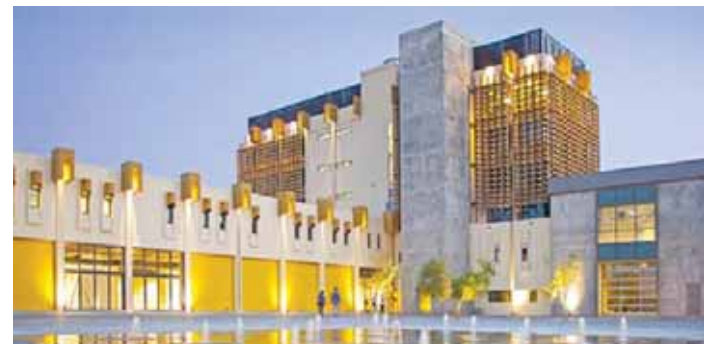
Fire Station artists' building in Doha.
