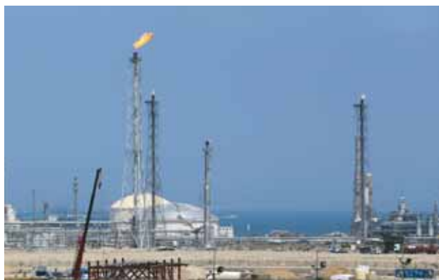
The Shuaiba oil refinery south of Kuwait City (file). KPC could restore its refinery output to normal levels in around two to three weeks. KPC has about 1.4mn barrels per day of refining capacity, its managing director for international marketing, Sheikh Khaled Ahmad al-Sabah, said.
