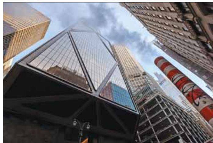
The JPMorgan Chase & Co global headquarters building in New York. JPMorgan has more than 550 bankers covering innovation economy clients globally - 200 of which were hired since 2023 - and works with over 11,000 startups and high-growth companies across 40 countries.
