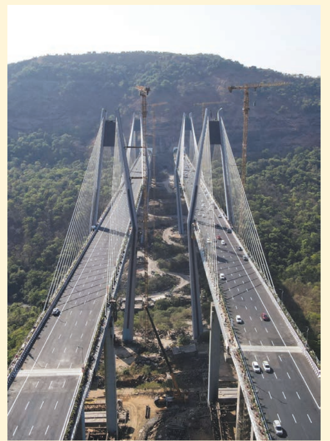
A drone view of traffic moving on the new Mumbai-Pune Expressway Missing Link project in Khopoli, India. (Reuters)
