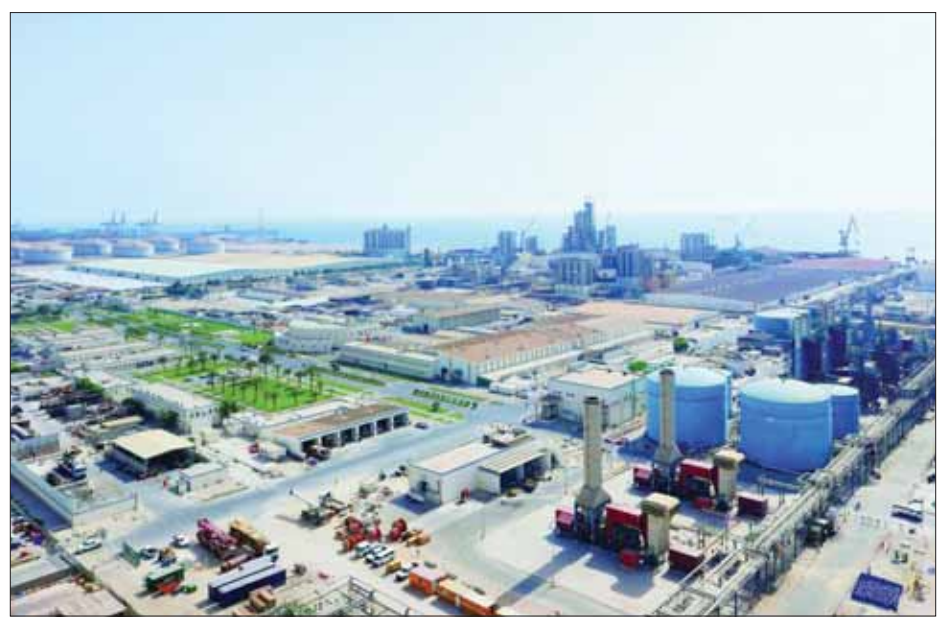
An aerial view of Qapco facilities in Mesaieed (file). Market heavyweight Industries Qatar (IQ) -- the holding group of Qatar Petrochemicals, Qatar Fertiliser and Qatar Steel -- has reported net profit of QR734mn; translating into earnings-per-share of QR0.12 at the end of first quarter (Q1) ended March 2026.
