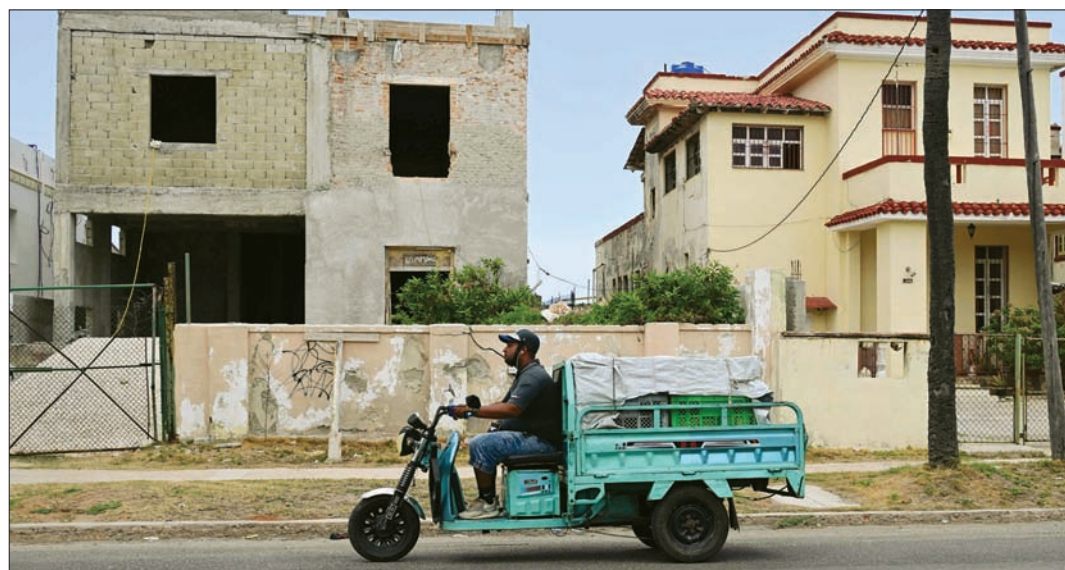
A tricycle goes past a house under renovation in a neighborhood of Havana. (AFP)
