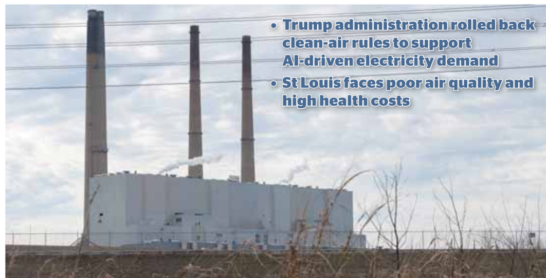
The Labadie power plant, outside of St Louis, Missouri, US. (Reuters)
