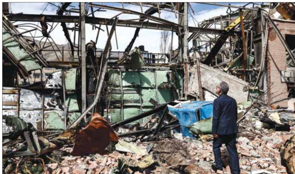
Iran's Minister of Science Hossein Simaee Sarraf inspects the damage at the research building of the Shahid Beheshti University, which was damaged by a strike, amid the US-Israeli conflict with Iran, in Tehran, yesterday. (Reuters)
