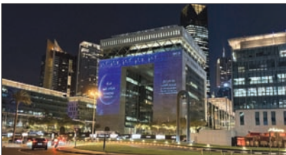
Exteriors of buildings in the Dubai International Financial Centre (DIFC), as banks step up precautions after Iran threatened Gulf banking interests linked to the US and Israel, in Dubai, yesterday. (Reuters)
