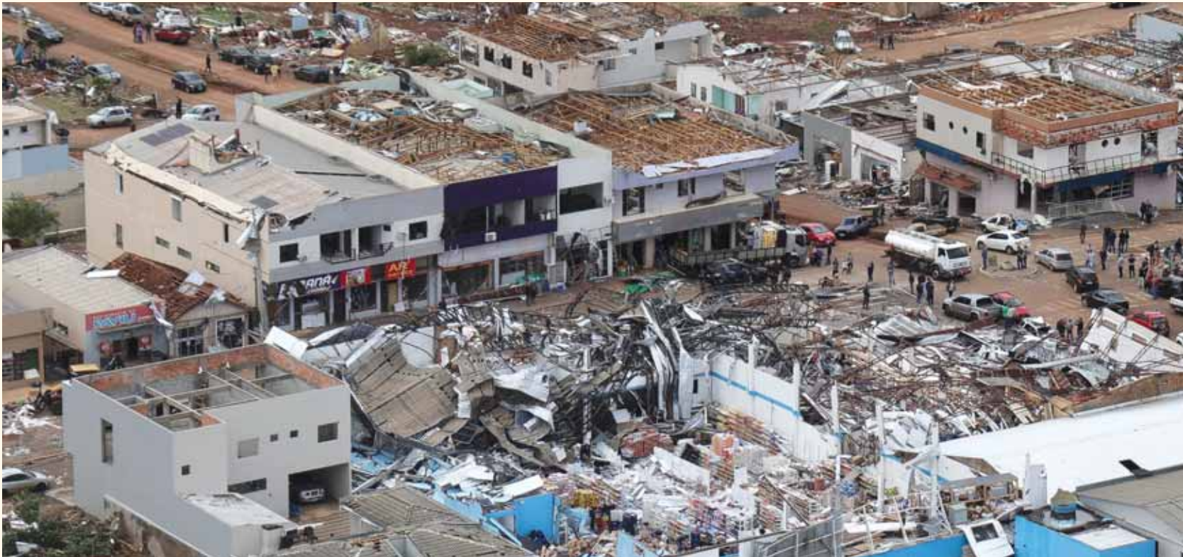
An aerial view shows damaged buildings after a tornado hit Rio Bonito do Iguacu, Parana state, Brazil, yesterday.
