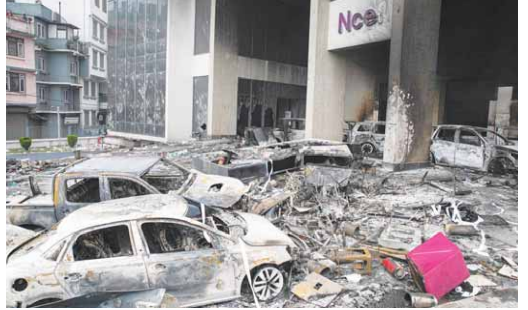
Charred vehicles lie amid the remains of the torched Ncell headquarter building, Nepal's leading mobile service provider, a day after it was set ablaze by protesters in Kathmandu yesterday.
