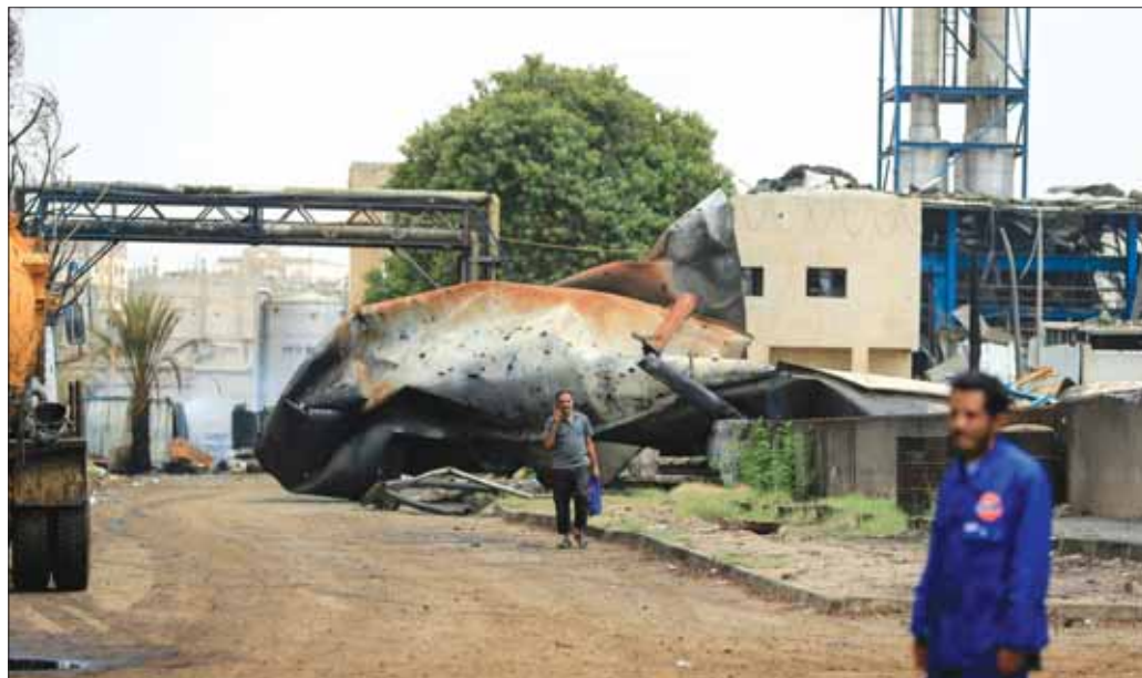
A man walks as another looks on at the site of an Israeli air strike that targeted the Haziz power station south of the Houthi-run Yemeni capital Sanaa, yesterday.
