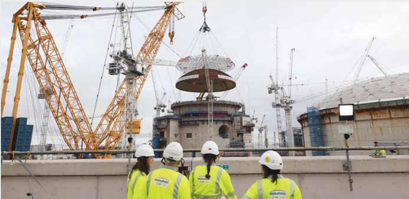
Media crews gather to witness the world's largest land crane 'Big Carl' lifting a 245-tonne domed roof onto Hinkley Point C's second reactor building at the Hinkley Point C nuclear power station near Bridgwater in southwest England, yesterday.
