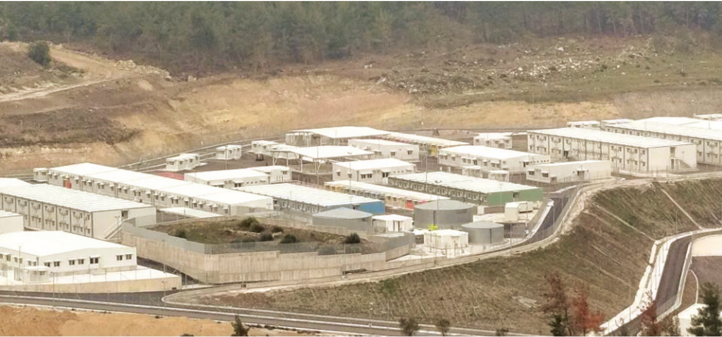
A view of the Closed Controlled Access Centre construction site in Vastria forest in Lesbos.
