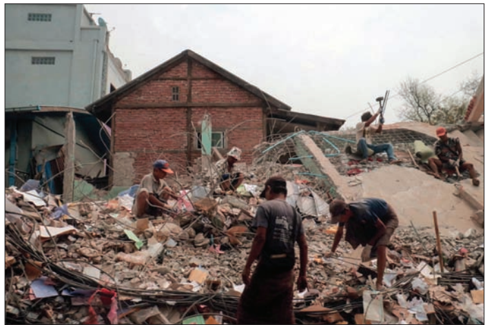
People sort through the rubble of a collapsed building in Mandalay.
