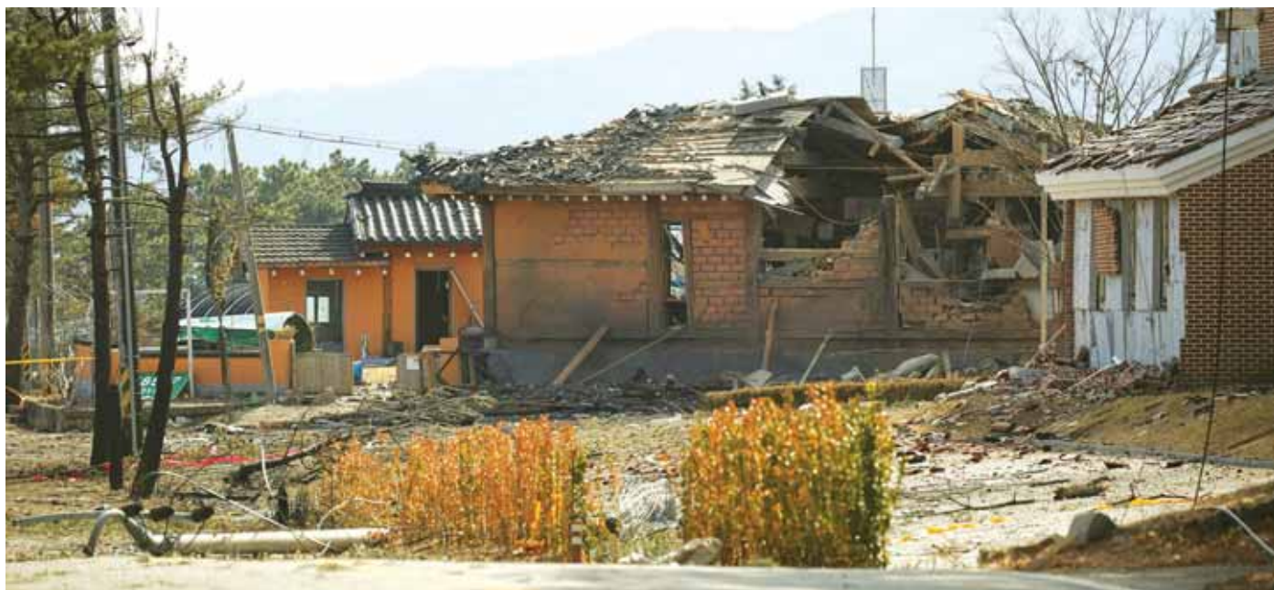
Debris lies near the damaged buildings after the accidental bombings in Pocheon, South Korea, yesterday.
