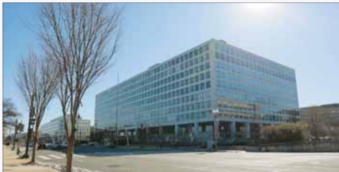
An exterior view of the Federal Aviation Administration headquarters in Washington. Aviation industry groups and union leaders called on the FAA to expedite upgrades to critical air-traffic control systems, as Elon Musk pushes SpaceX's Starlink as a solution for modernisation.
