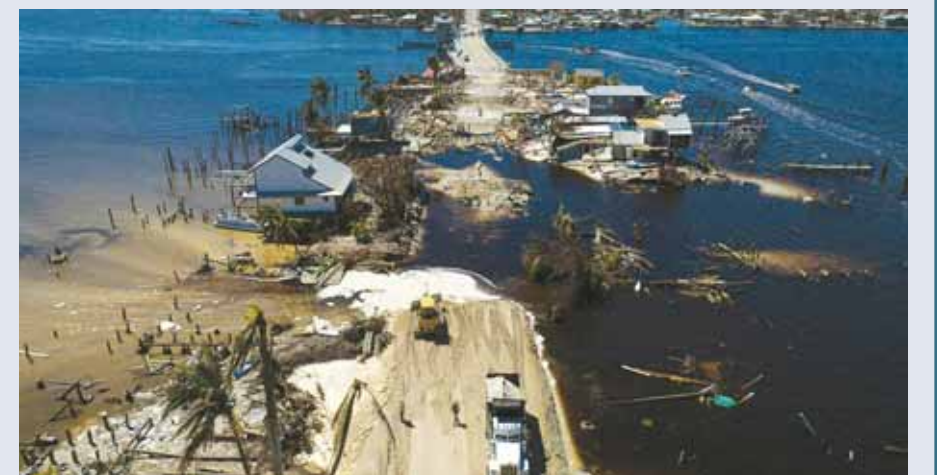
FILE PHOTO: An aerial picture taken on October 3, 2022 shows a dump truck dumping its load during emergency repairs to restore road access in the aftermath of Hurricane Ian in Matlacha, Florida. (AFP via Getty Images)
