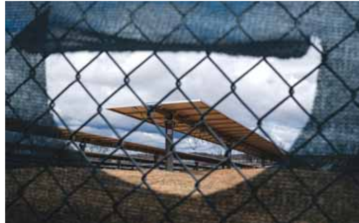
Solar panels stand on sandy soil located on Dave Duttlinger's farmland that he leased to Dunns Bridge Solar LLC in Wheatfield, Indiana. (Reuters)
