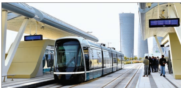
Each Lusail Tram station contains a customer information centre, Travel Card vending machines, live digital service updates, separate male and female prayer facilities and restrooms that cater for people with mobility impairments.
