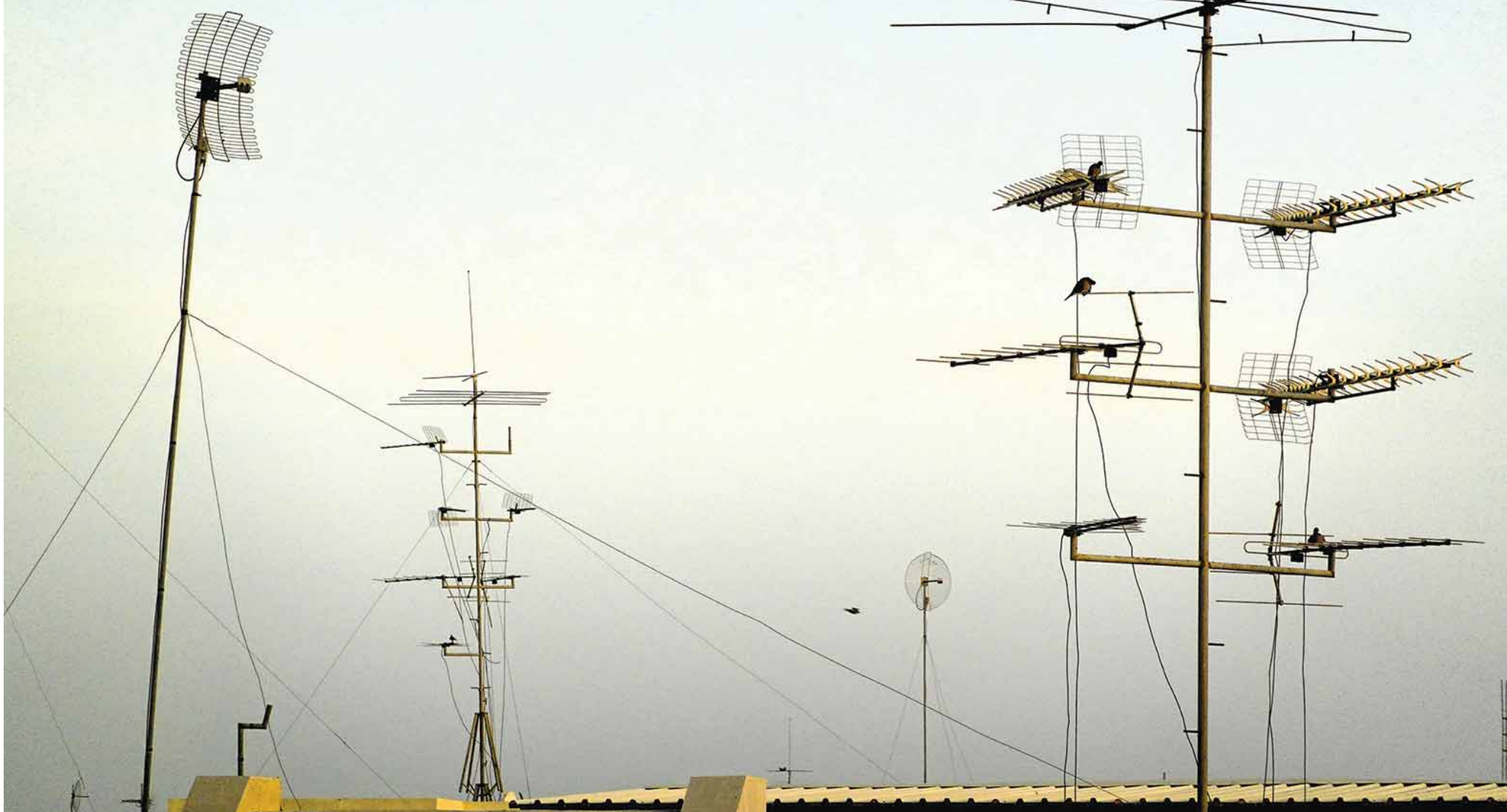
The Yagi-Uda antennas, remnants of the early days of television, continue to be seen across many Doha rooftops despite becoming redundant decades ago with advances in broadcast technology. These antennas, developed by Japanese inventor Shintaro Uda and his colleague Hidetsugu Yagi in 1926, were in use all over the world for several decades. In Doha, these forgotten equipment serve as bird perches. PICTURE: Gulf Times news editor Bonnie James.
