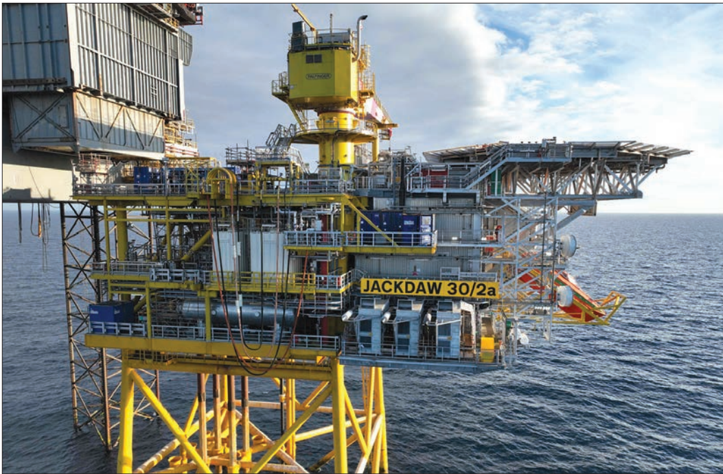
The Jackdaw gas production platform in the North Sea, 250km east of Aberdeen, Scotland. Britain on Wednesday approved the Jackdaw North Sea gas field, ending years of legal and political wrangling as the Labour government seeks to balance its climate goals with energy security concerns.
