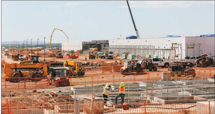
Data centre buildings are under construction in Abilene, Texas. The artificial intelligence boom, increasingly acknowledged at the Federal Reserve as helping drive inflation, has left central bankers faced with cooling the rest of the economy to lower price pressures amplified by an industry of marquee names like Amazon, Apple and Anthropic considered immune to rate hikes.
