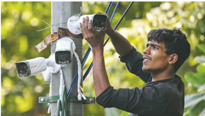
A worker installs CCTV surveillance cameras near the Jantar Mantar protest site in New Delhi yesterday on the eve of the planned protest by the Cockroach Janta Party. (AFP)
