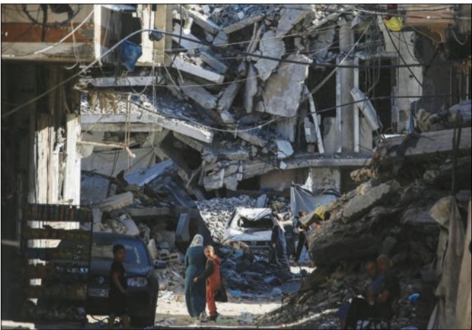
Palestinians walk along a street lined with destroyed buildings at the Jabalia refugee camp in the northern Gaza Strip. (AFP)
