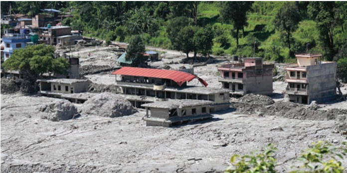
A general view shows damaged houses covered in sludge in the aftermath of flash floods at Trishuli in Nuwakot district. (AFP)
