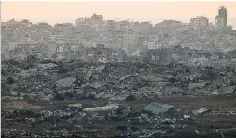
Destroyed and damaged buildings remain in Gaza. (Reuters)
