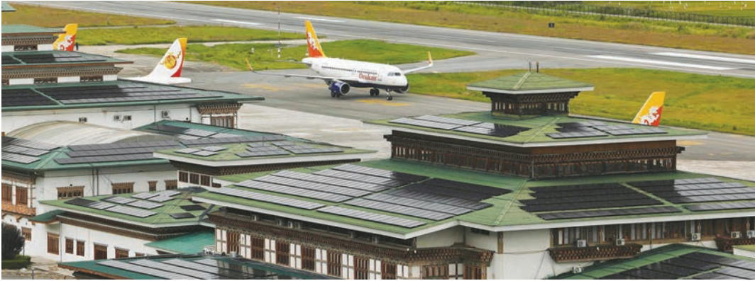
This photograph shows solar panels on rooftops of buildings at Paro International Airport in Paro city. (AFP)
