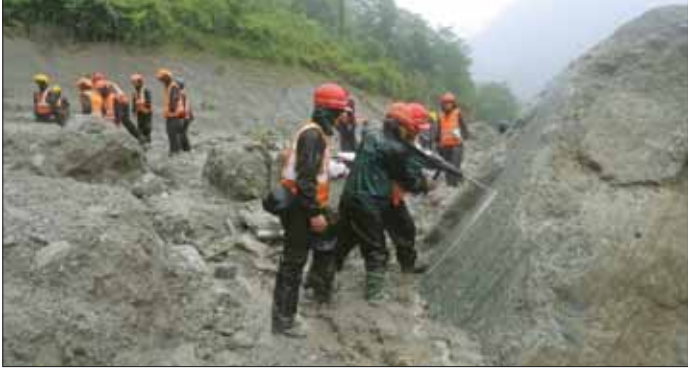
An undated handout photo of rescue workers taking part in a rescue operation near the tunnel of the Trishuli 3A Hydropower Project, following deadly flash floods and mudslides, in Rasuwa, Nepal. (Reuters)
