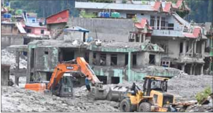
An excavator helps people to collect some of their belongings from their house at Trishuli, in Nepal’s Nuwakot district, yesterday. (AFP)
