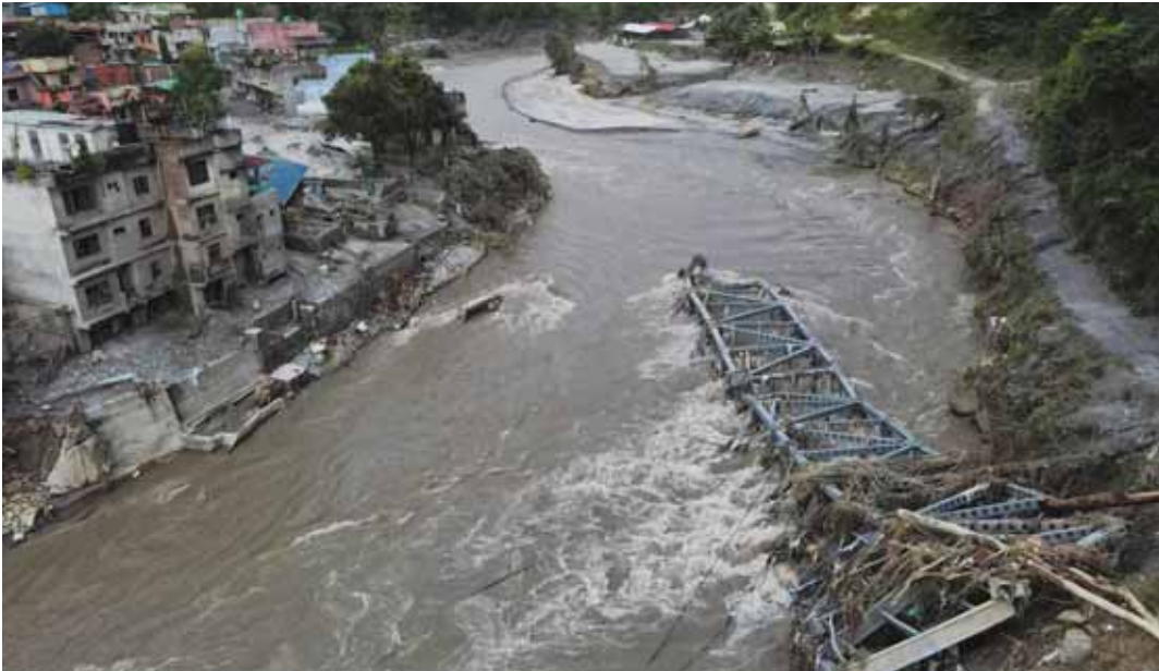
A drone view of a broken bridge and damaged houses after the flash floods and mudslide, at Devighat, Nuwakot district, yesterday. (Reuters)
