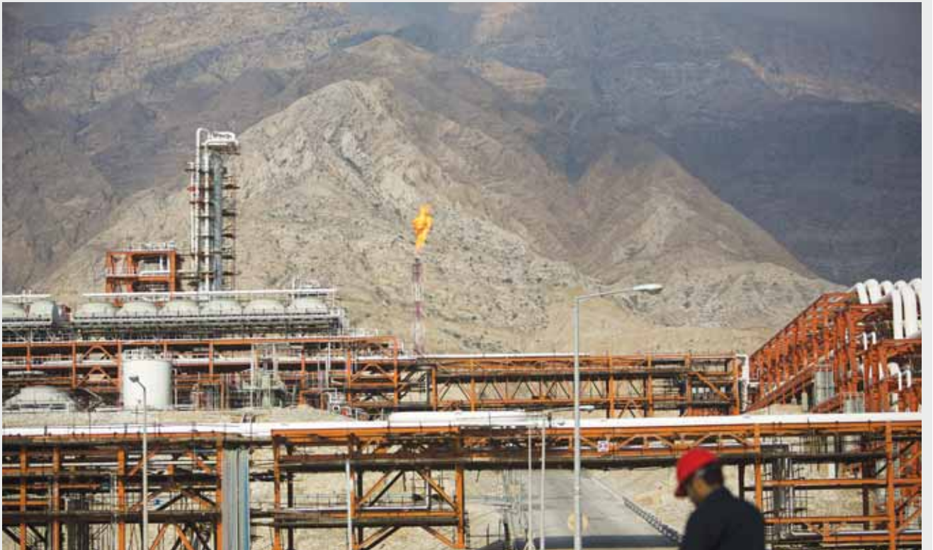
An Iranian worker walks along the phase 15-16 of the South Pars gas field facilities in the southern Iranian port of Assaluyeh on the shore of the Gulf (file). Around 40% of the South Pars gas field capacity damaged during the war is back in production, Iran's Deputy Oil Minister Ahmed Zeraatkar said on Thursday, according to Fars news agency, reports Reuters. South Pars is the world's largest offshore natural gas field. Meanwhile, Iran's oil sales and deliveries in "distant waters" continue despite reduction, Iran's Oil Minister Mohsen Paknejad said on Thursday according to state media.
