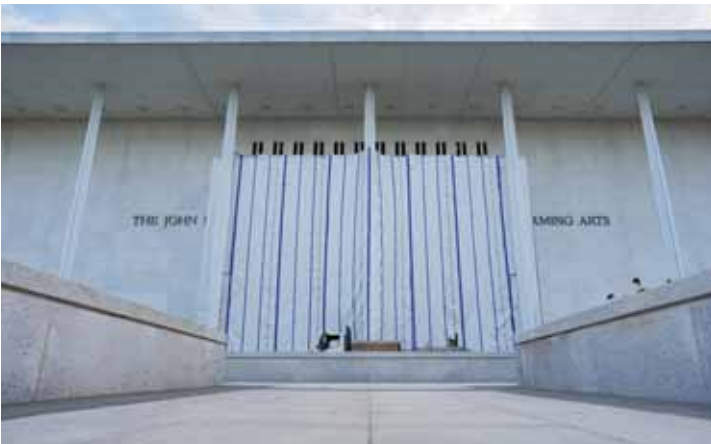
A tarp covers the facade of the John F Kennedy Memorial Center for the Performing Arts, following a federal judge's order to remove Donald Trump's name, in Washington, DC. (Reuters/File Photo)
